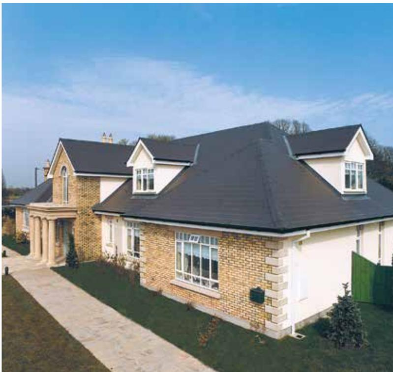
The Rustic, is a rectangular textured fibre cement slate with square edges which give the appearance of traditional natural slate to all types of roofs. The slates have a thickness of 4mm (nominal: 4.1 mm).
